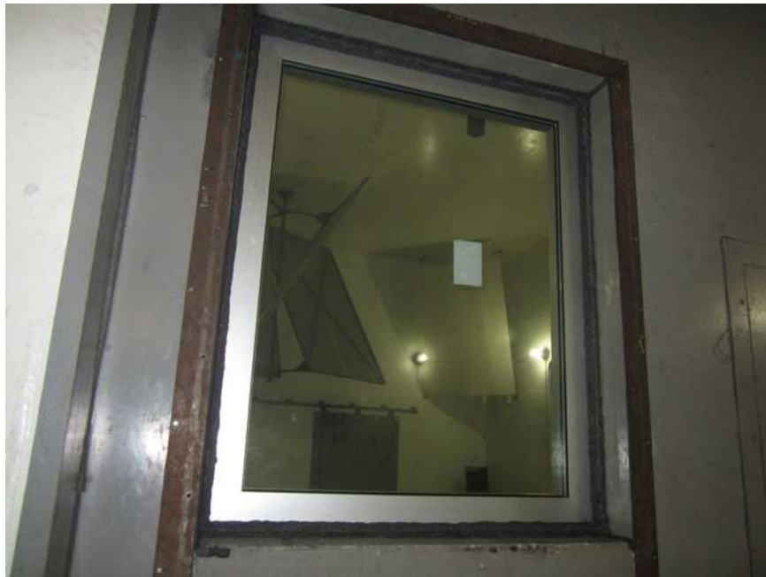
Source Room View of Installed Specimen
