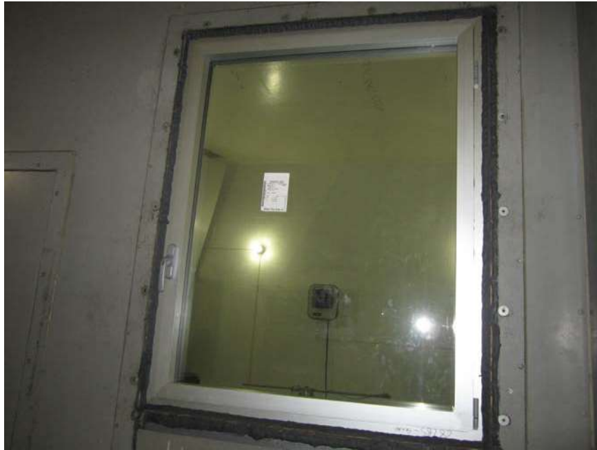
Receive Room View of Installed Specimen
